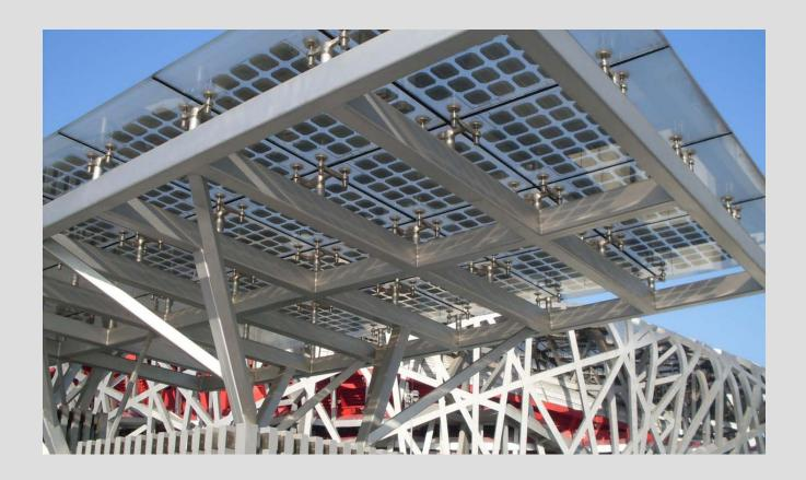
BIPV modules use double sided low iron tempered glass with solar cells laminated in between. BIPV modules are ideal for roofs, skylights and/or facades. BIPV modules can not only be used as a part of construction material for a building, but also as a source of electricity.
