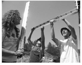
PV array assembly. The mounting pole is short enough to facilitate assembly without mechanical assistance.
