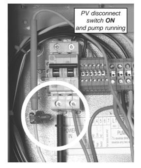
Remove one array wire and re-make the connection **THROUGH** your meter. Probe connections must be secure. A clamping device is helpful (split bolt is shown as an example).
