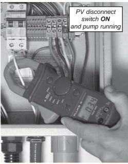
DC clamp-on meter must be zero-set first
