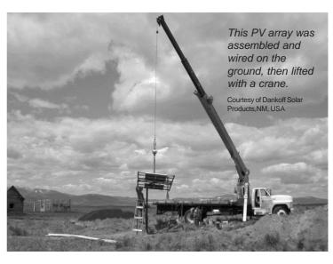
PS600 HR04-300Wp system in Colorado, USA, installed by students in a solar pumping class.
